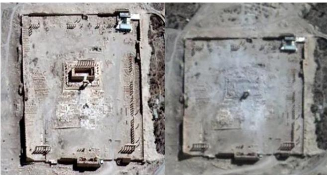
Satellite images of the Temple of Bel, Palmyra, before (L) & after (R) its destruction by Isis in Sep 2015
